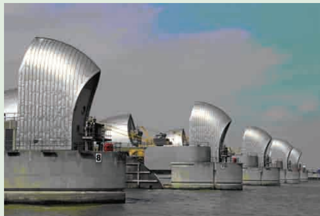
Box Figure 6.2: The London Barriers are the centerpiece of today's Thames Tidal Defenses that protect London and the Thames Estuary corridor where a significant proportion of England's wealth is produced (1.25 million people live and work in the flood risk area). The system provides at least a 1:1000 per year protection (to 2070). The system allows for a combination of risks (high tide/surge/freshwater floods). It comprises 9 tidal barriers (including the Thames Barrier), as well as, 35 major gates, 400 minor gates and over 300 km of tidal walls and embankments.
